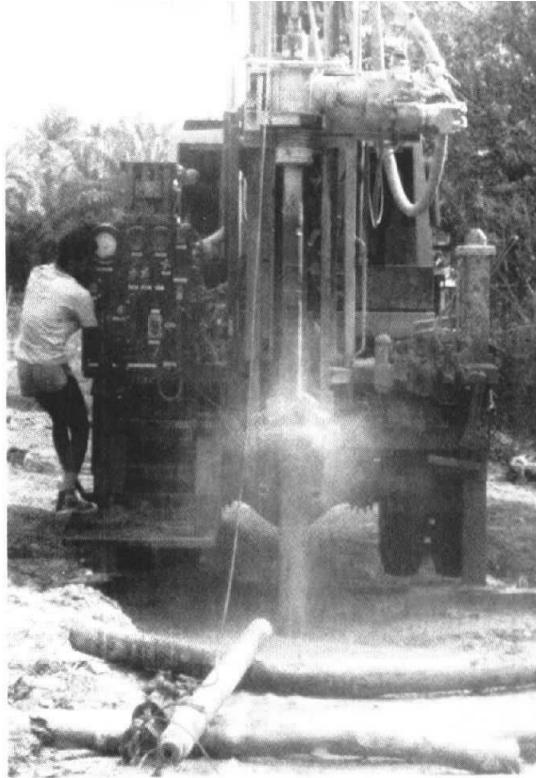
Drilling a water well in Okposi region of southern Nigeria, east of Niger River Courtesy UNICEF (Maggie Black)
